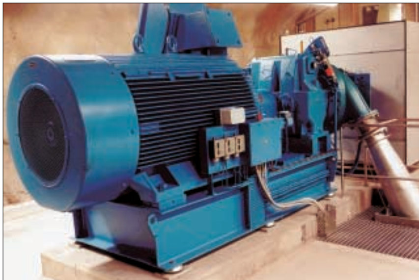
Fig 1. High pressure compressor mounted on Novibra type RA.
